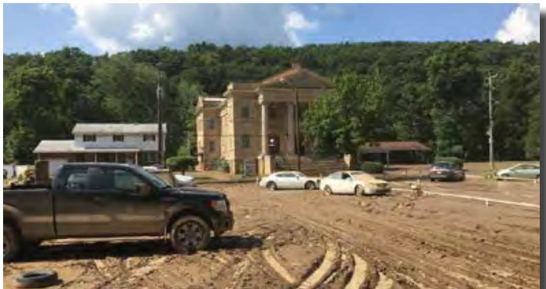
Clendenin United Methodist Church immediately following the flood
